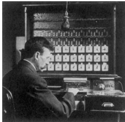
■ Fig. 1.13 Tabulating machines. The Hollerith Tabulating Machine was an early data-processing system that performed automatic computation using punched cards. (Photograph courtesy of the Library of Congress)
